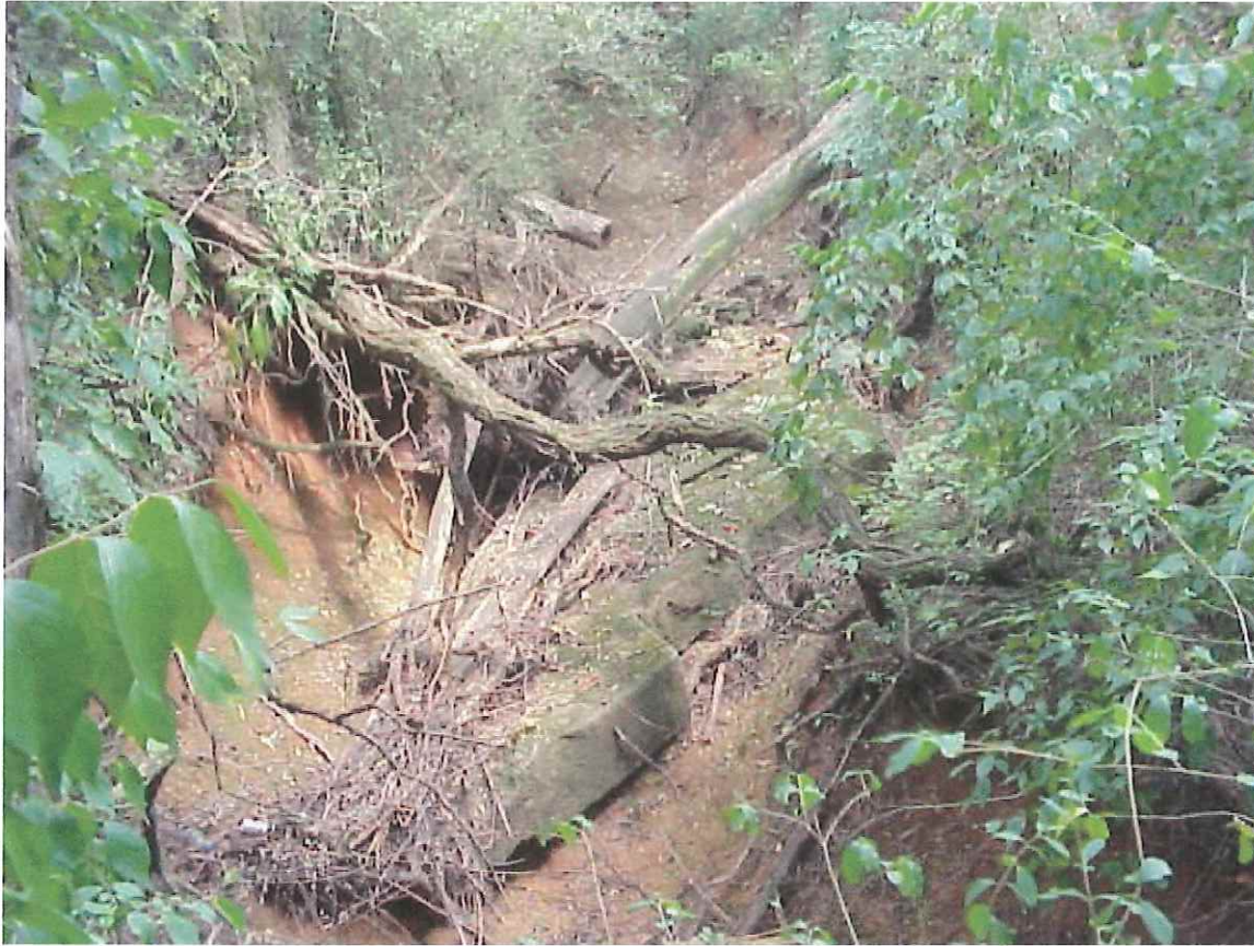
Figure 7-5. Briar Glen priority area– Erosion region with debris (looking upstream)
